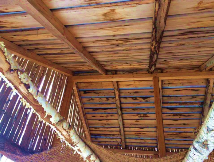
Figure 34. Roof boards for coverage
