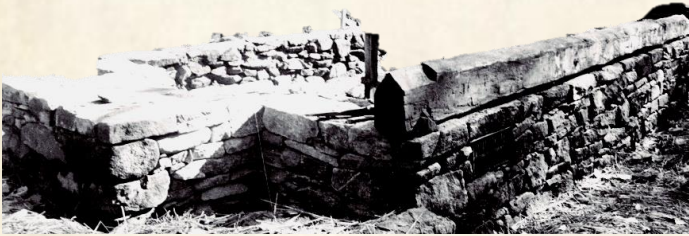
Figure 22. Stone foundation & V-shaped log
