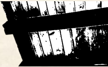
Figure 29. Shiplapped ceiling
