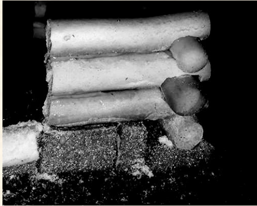
Figure 20. Log notching on round-shaped logs
